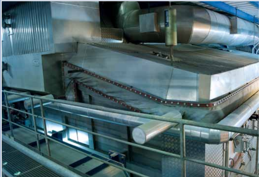
Multilayer expansion joint bellows, type GB300 as a seal between the grate and boiler in a waste incineration plant
